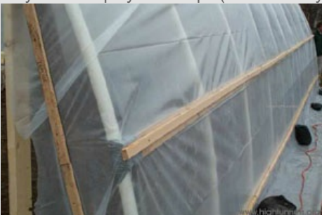
Figure 10. Poly attachment to hip board using one furring strip. This method is less secure than others since poly tends to tear at the screws.
