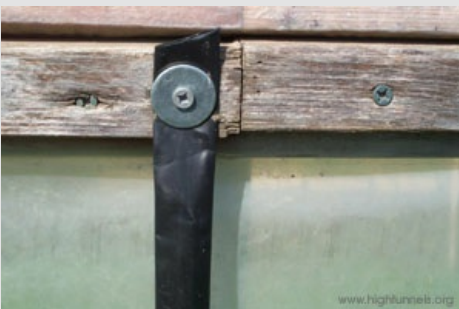
Figure 13. A drip tape strip from hip board to base board at each hoop can keep side walls from billowing.
