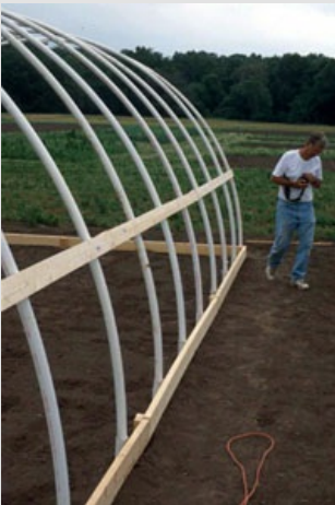
Figure 7. Hip board in place.
