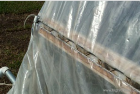
Figure 12. Poly attachment to hip board using wiggle wire.
