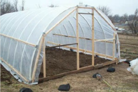
Figure 9. Tunnel showing end wall design at Full Circle Farm, Kansas City, Kansas.
