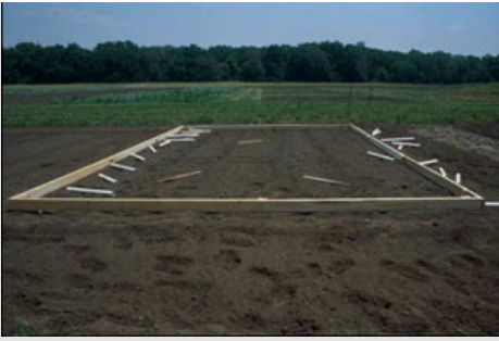
Figure 1. Baseboards laid-out ready for ground post installation.
