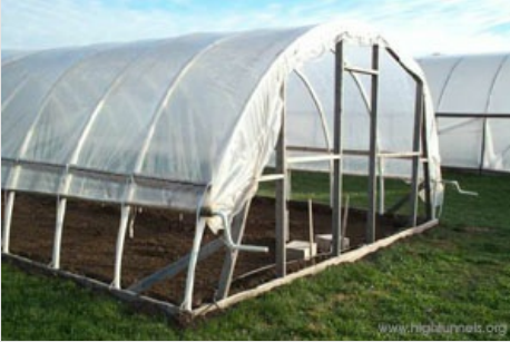
Figure 8. Tunnel showing end wall design at K-State Research and Extension Center, Olathe, Kansas.
