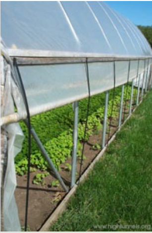
Figure 11. Picture showing the 2-furring strip method of attaching poly to the hip board.
