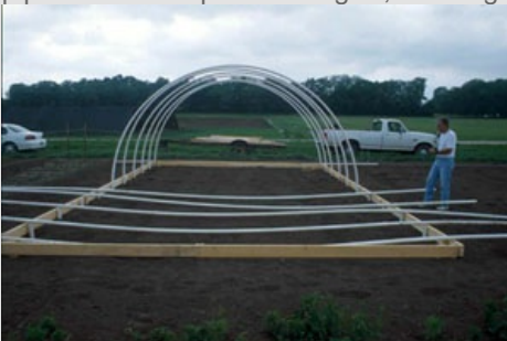
Figure 4. Hoops being placed in ground posts.
