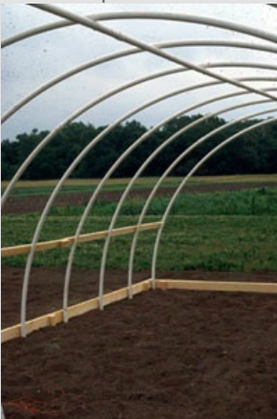
Figure 6. Tunnel with purlin and hip board in place.
