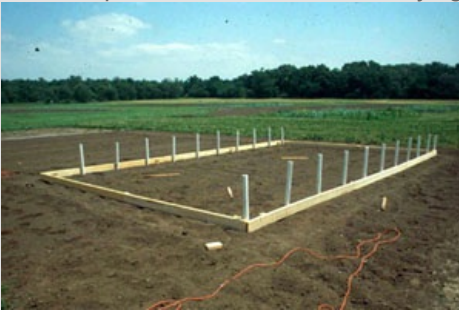
Figure 2. Ground posts ready to be driven in.
