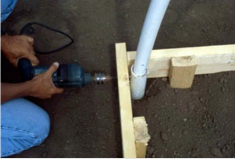
Figure 5. Drilling through baseboard, ground post and hoop. Carriage bolts will hold hoop in place.
